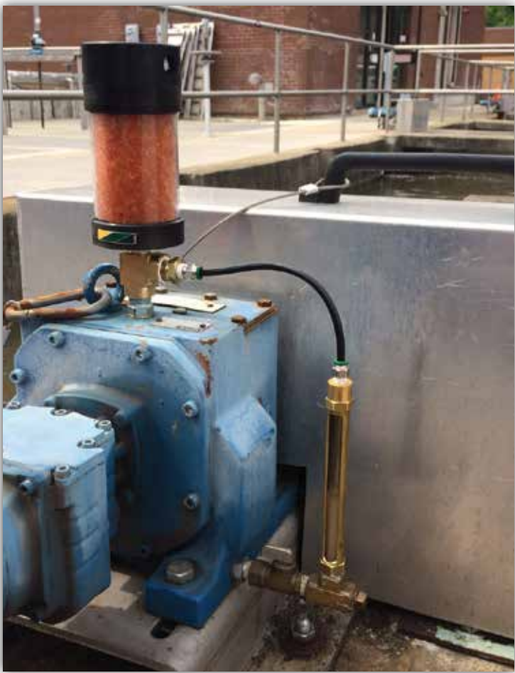
Closed system liquid level gauge with pressure balancing line.
