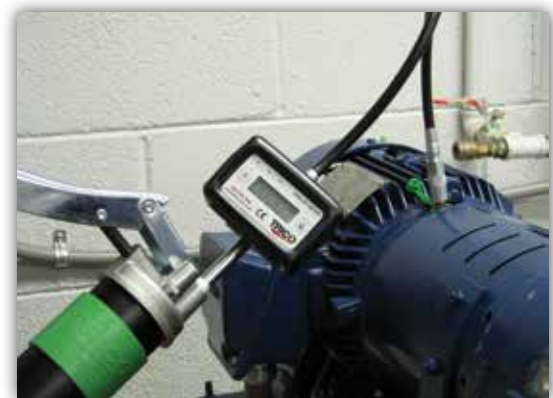
Grease meter being used with Spectrum Grease Identification Products to ensure the right grease goes into the right piece of equipment.
