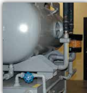
Watchdog Breather installed on a hydraulic reservoir
