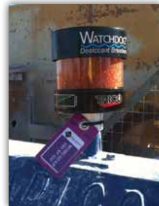
Spectrum Tag on a Watchdog Desiccant Breather
